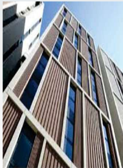
GRC with V Groove / Open Joint
