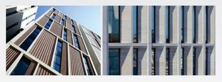
GRC WITH V GROOVE / OPEN JOINT
